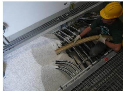
Picture F: Cable Cellar Suction
