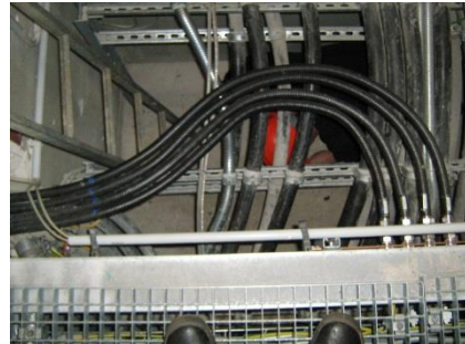
Picture D: Cable Cellar Pre Filling
